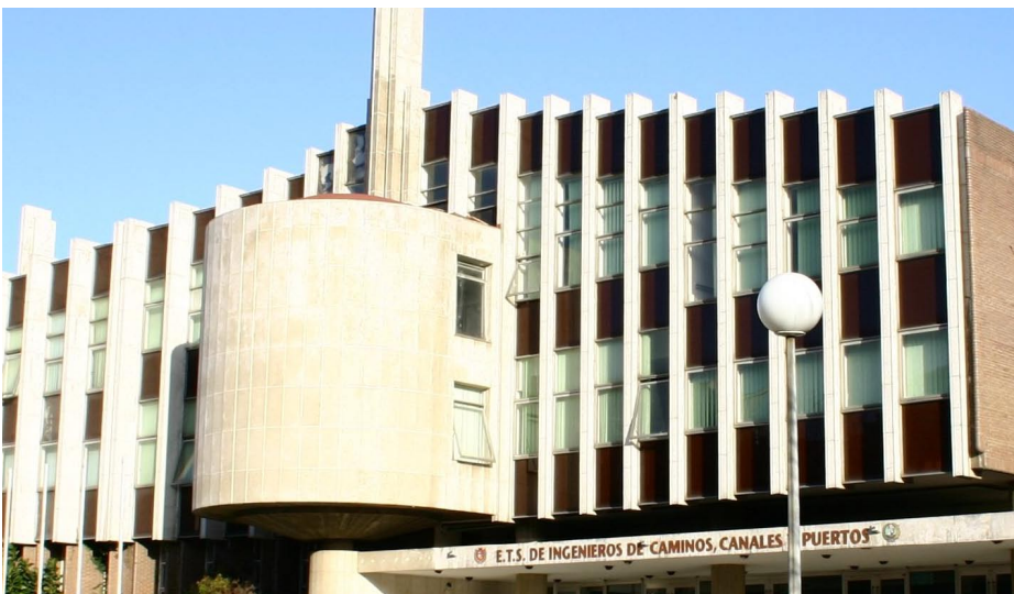
School of Civil Engineering in Santander
